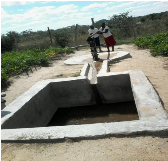
Plate 4.7 Mutsiba Garden borehole and 2,400 litres capacity water trough
