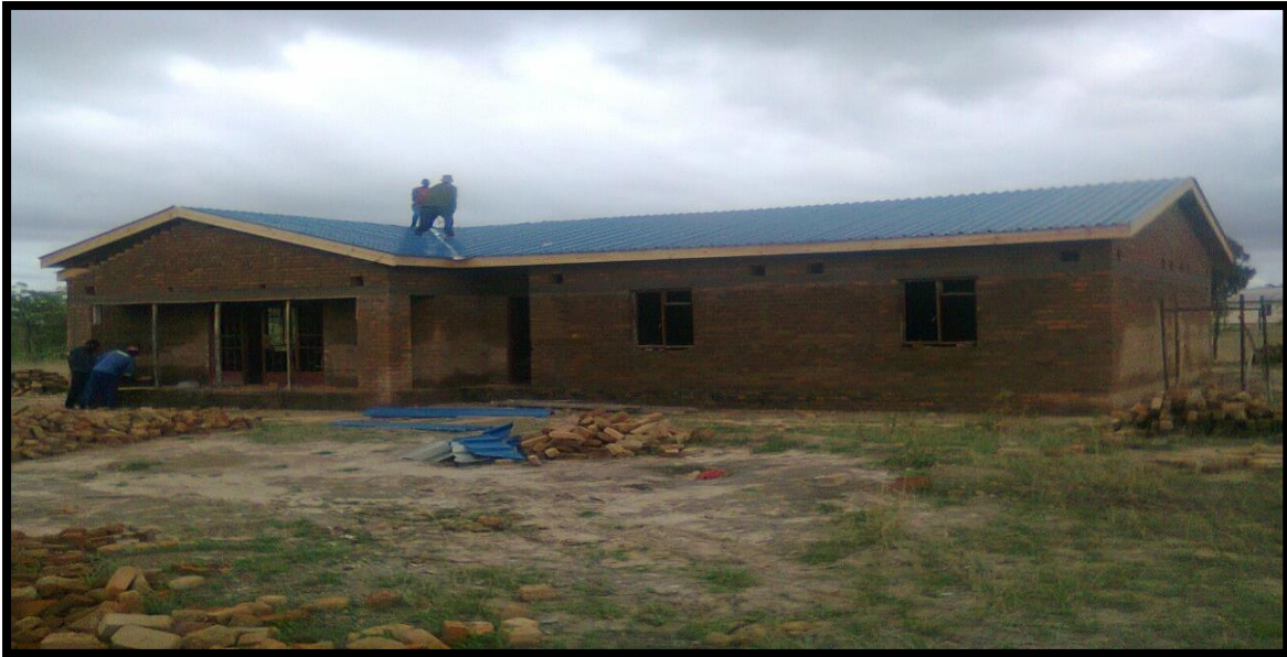
Figure 2 F.I.F Children’s Home Bondamakara Mtoko, 2nd house under construction
