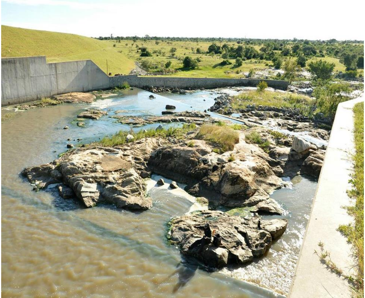
Plate 4.1 :Insukamini Dam (Ward 8) in Lower Gweru
