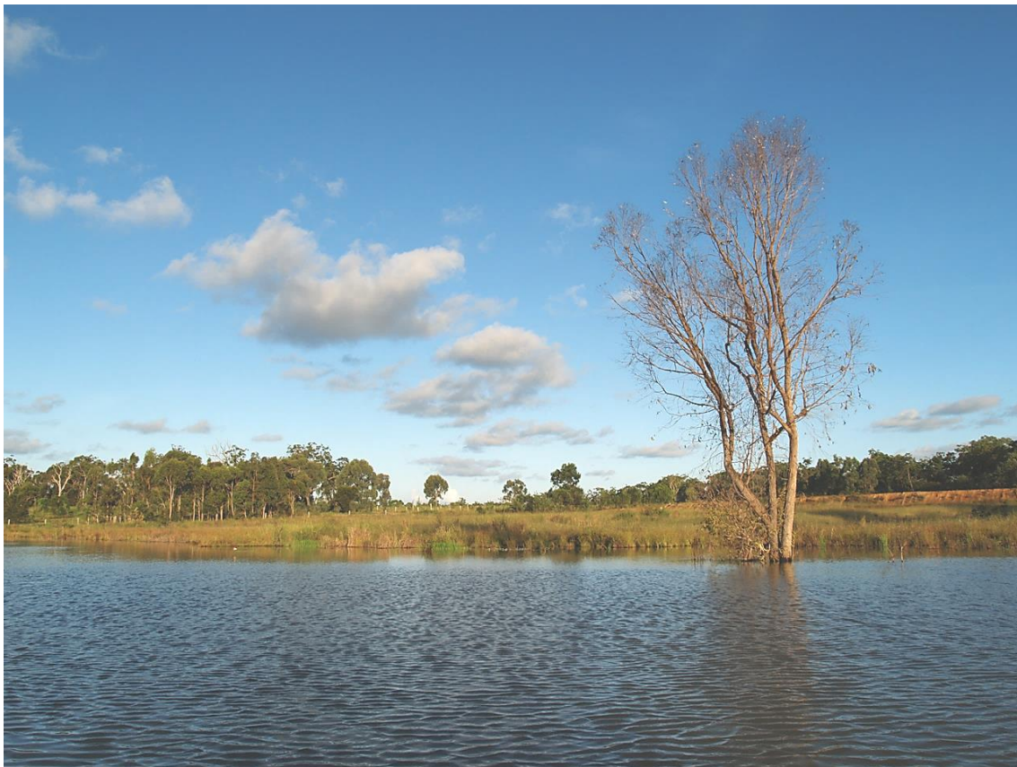
Plate 4.5 :Bembeswana Dam in Kabanga –Chiundura Source:Field Survey 2018
