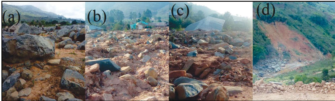
Figure 4.13: Homesteads at Kopa completely destroyed and covered by rocks
