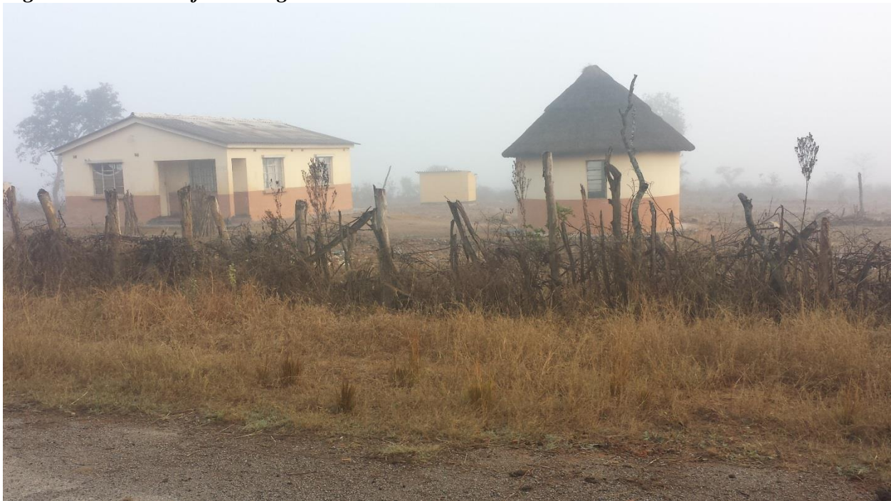
Figure 13: Picture of houses given to the relocated households
