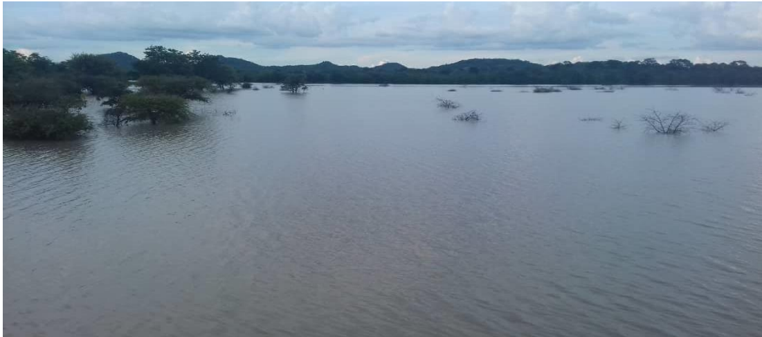
Figure 9 SHOWS RECONSTRUCTED MANYANE DAM IN MANYANE VILLAGE
