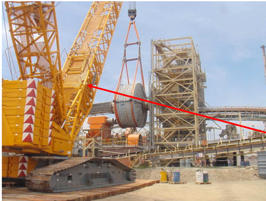
Plate 4.3: 600t Crane lifting sag mill. Source: Primary data.
